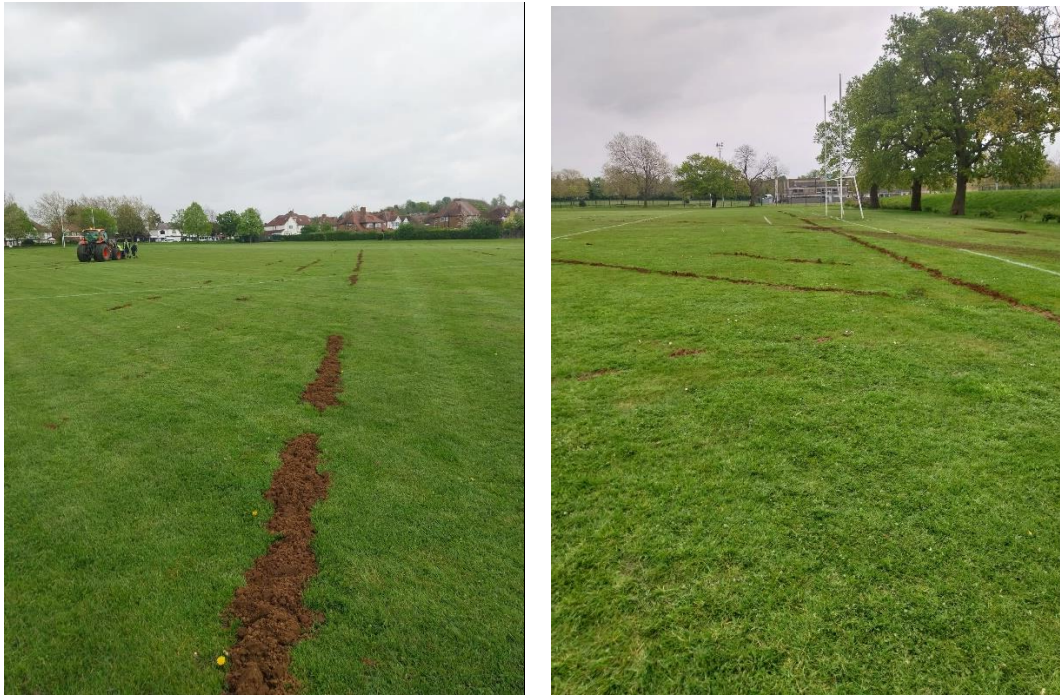
Figure 16 Image of Vale Farm Gaelic Pitch - Drain lines being filled with top soil
